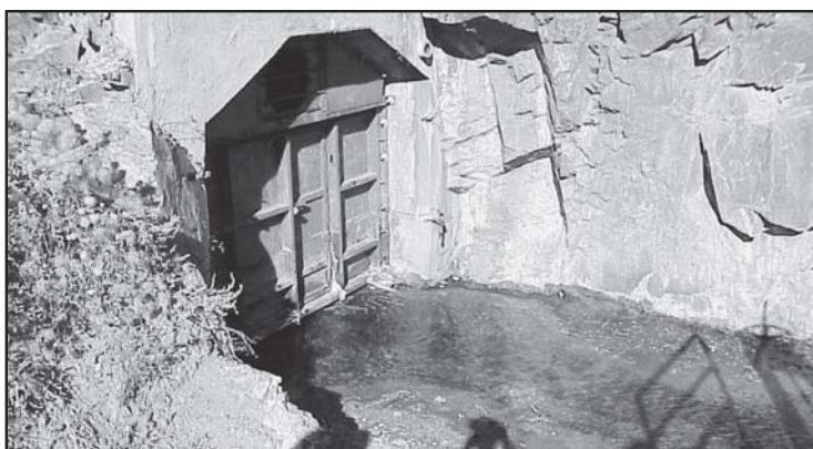
FIGURE 1.3 The Argo Tunnel near Idaho Springs, Colorado, typically produces water flow rates ranging from 200 to 300 gpm, depending on the season of the year. The pH ranges between 2.7 and 3.2, and the water contains high concentrations of zinc, iron, sulfate, cadmium, copper, and manganese.
